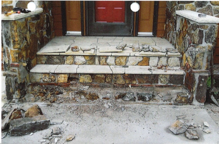
Front porch being repaired in 2010
