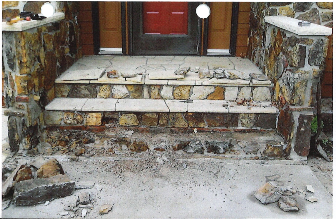
Front porch being repaired in 2010
